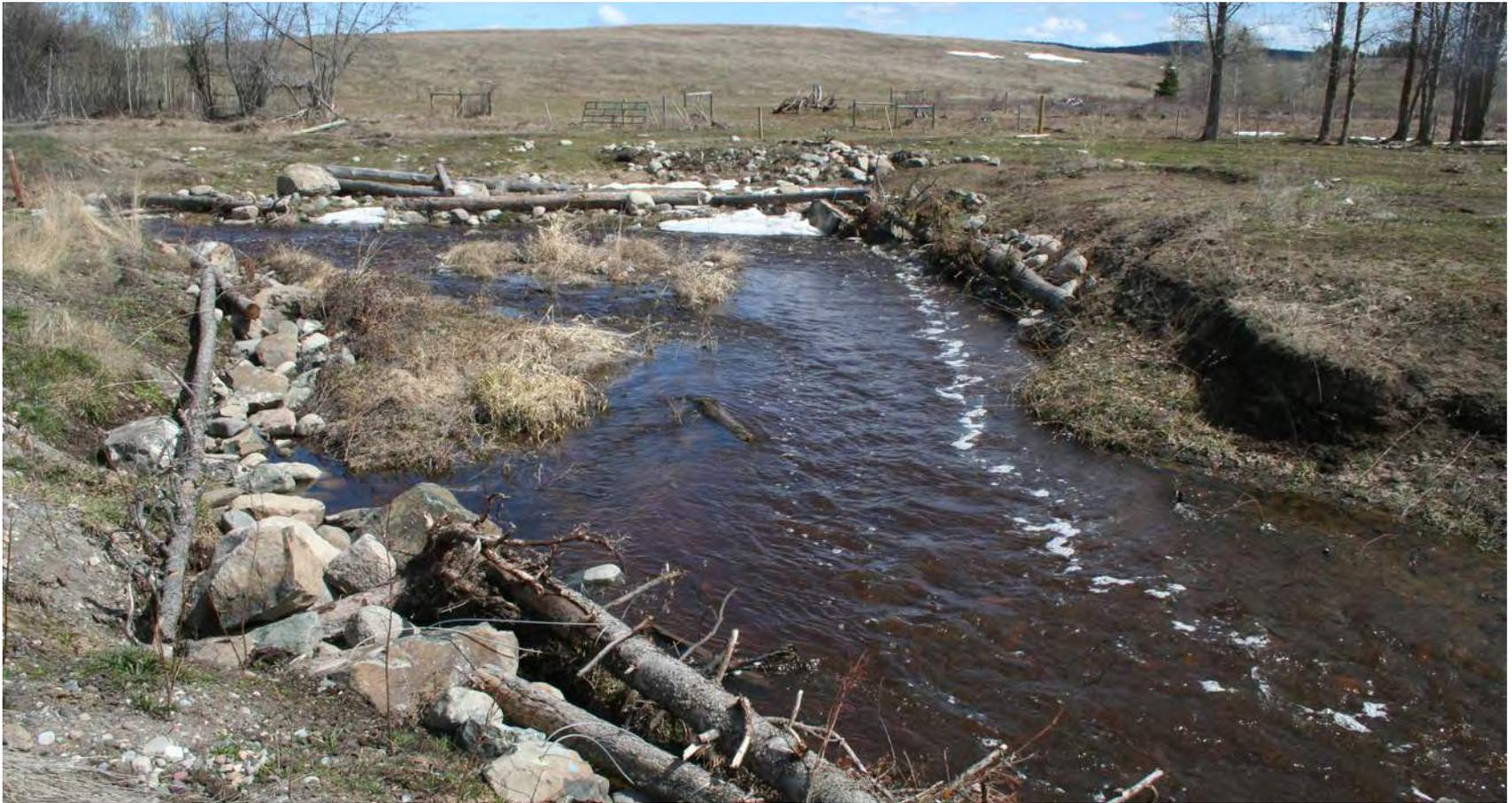
This section of Murray Creek was rehabilitated to reduce erosion and silt moving downstream to the Nechako River. It also improved the habitat for trout to spawn.
