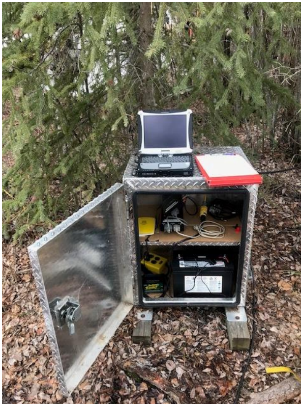
Photo 4: One of the telemetry station system upgrades that occurred in spring of 2021 (Photo by Ian Spendlow).
